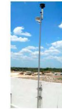
Figure 4. Mini-tower installed in the opposite side of the roof supporting an air temperature and a wind sensor
